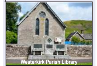
Westerkirk Parish Library
