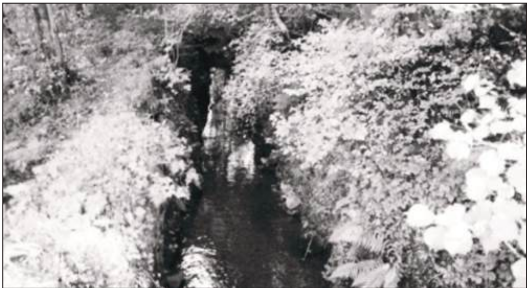
Part of the dam at Hollows Mill
