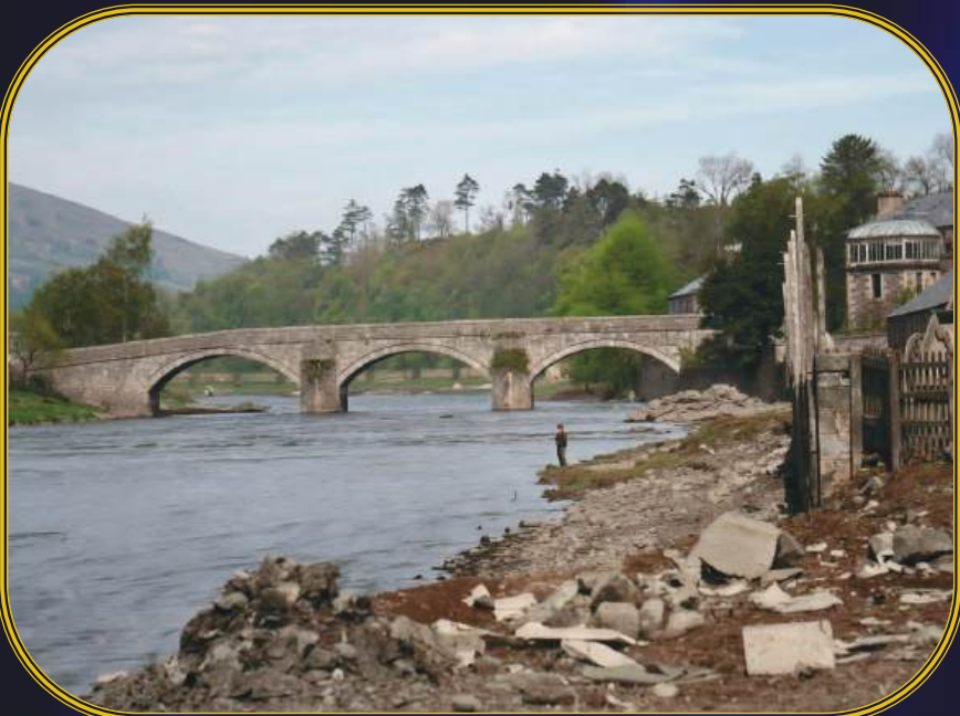
Langholm Bridge from Boatford 1868
