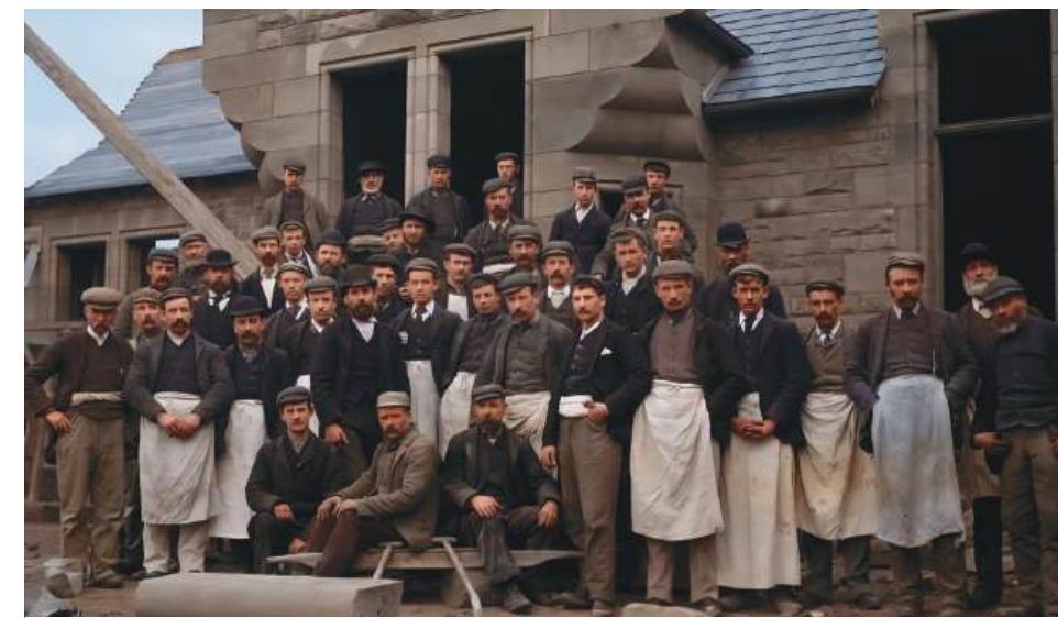
Construction of the Thomas Hope Hospital - 1896
