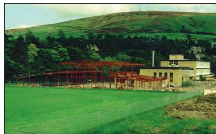
2001 saw the erection of the new Langholm Primary School...
