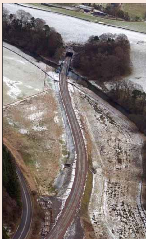
Electrification of Borders Railway route begins in March
