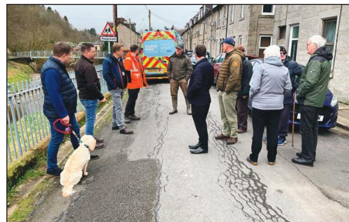
A meeting with roads engineers was originally held on Caroline Street on 27/02/24 to address the concerns about the safety of the structure of the street
