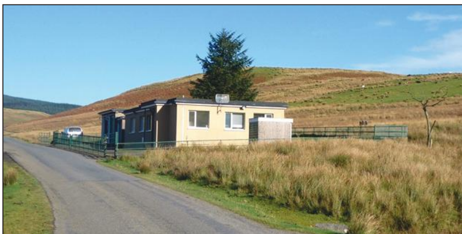
Eskdalemuir Seismological Station
