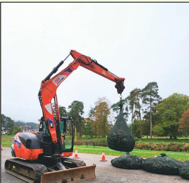
BEAR Scotland's crane on the Kilgreen with the bags of rock
