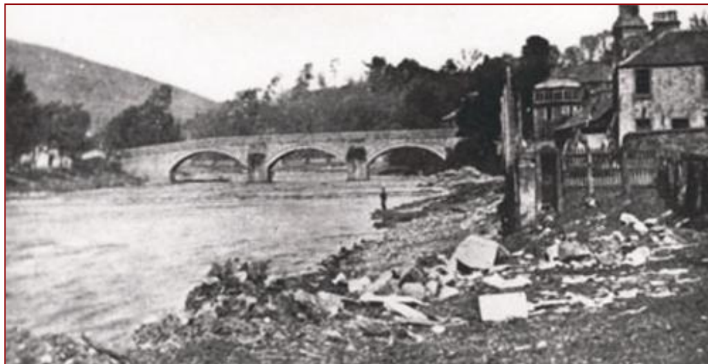
A very old, picture of Langholm Bridge with stone parapet. Thomas Telford was an apprentice on this bridge. Built by Langholm firm J Hotson - Photo Langholm Archive
