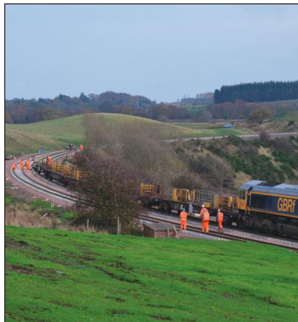
Track laying on the Borders route in 2014
