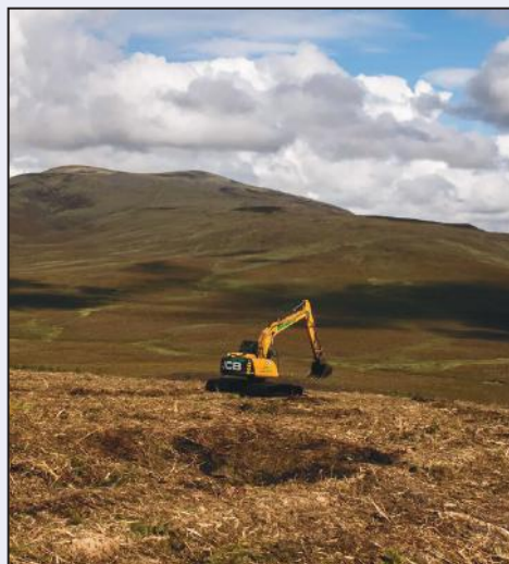
Peatbog restoration by Forestry and Land Scotland
