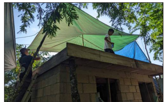
BEFORE & AFTER: Construction almost complete
