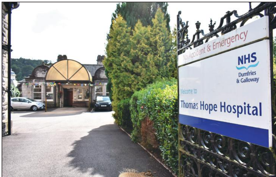
The Right Care, Right Place programme will be linked to the Murtholm development and the reinstatement of services in Langholm's Thomas Hope Hospital
