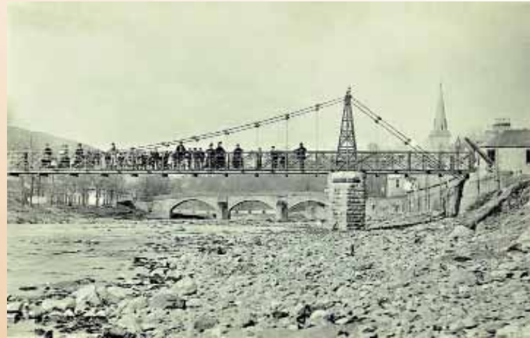
The re-built Boatford Bridge
