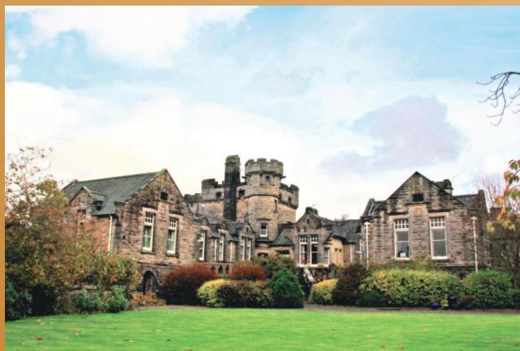
The front elevation of the Thomas Hope Hospital
