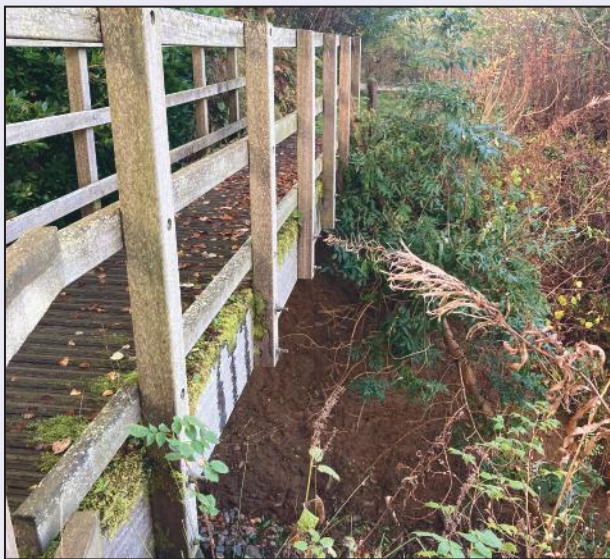
Gaskell's walk bridge is perched on precarious ground and left its location
